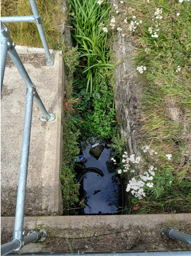
Watercourse immediately d/s of overflow
