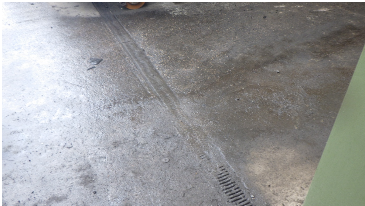
Drain across new depollution building.
