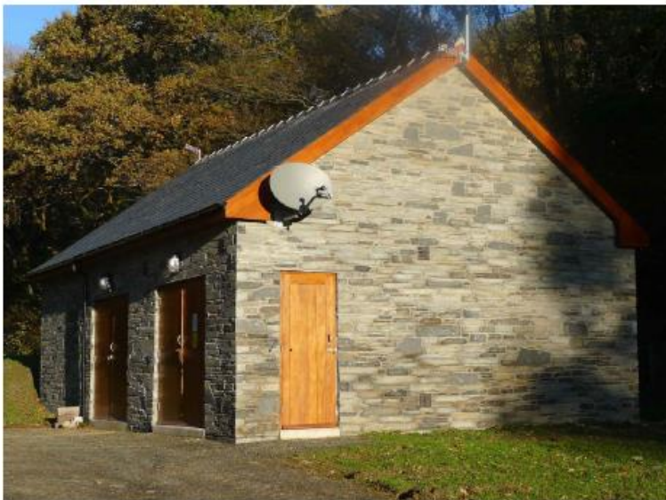
Example Power House Building Style Micro Hydro, 375kW Cadair Hydro
