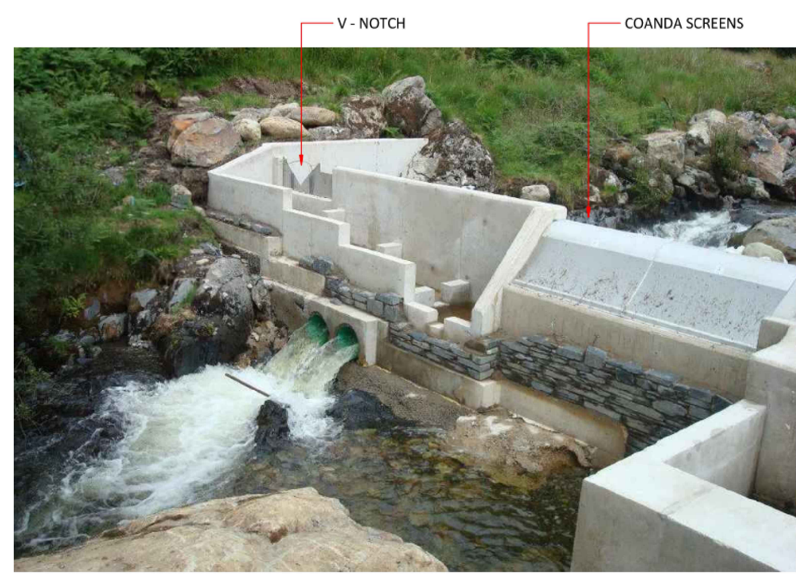
WEIR: Micro Hydro, 375kW Cadair Hydro (150m head, 300l/s, pelton turbine), operated by Dragon Hydro www.dragonhydro.com Photos: Jonathan Bensted
