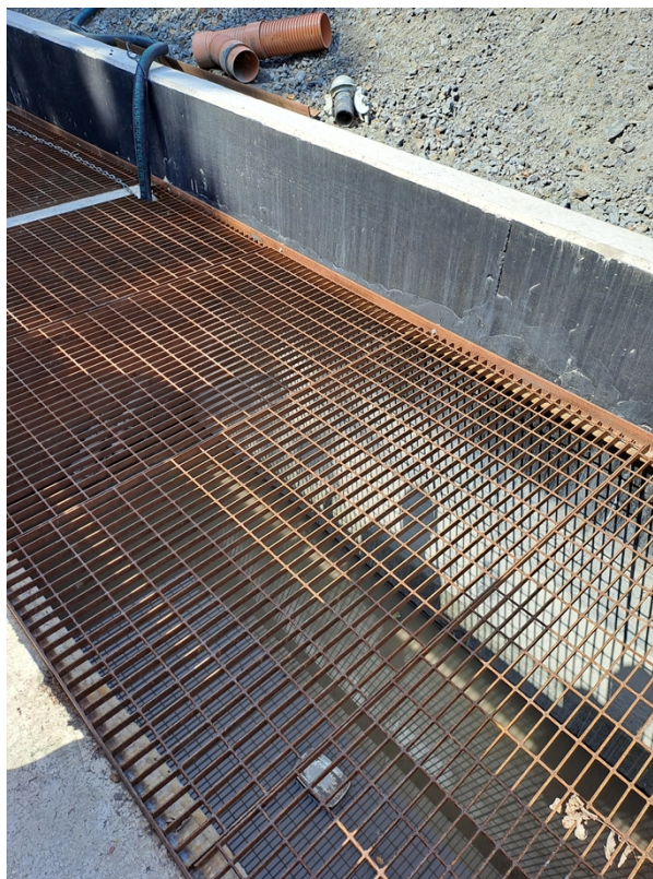
Figure 8 – The new final catchment weir as observed during the visit.
