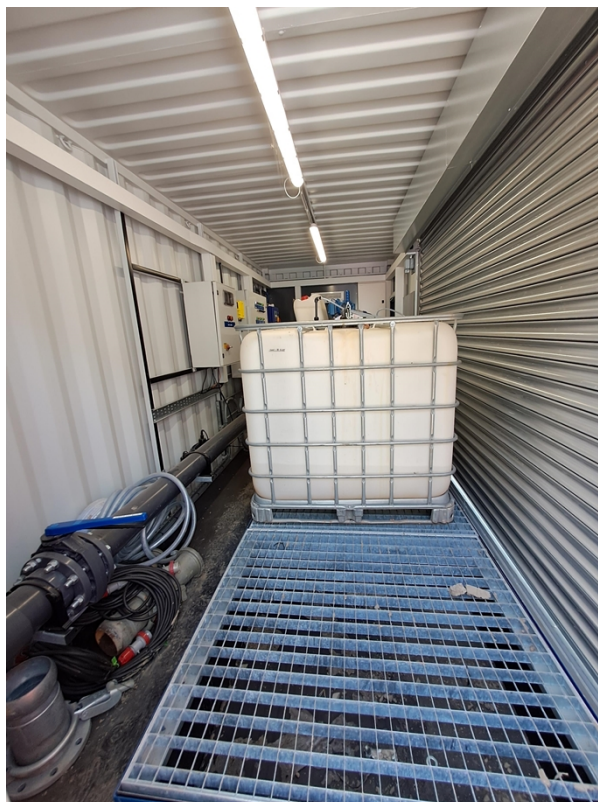
Figure 7 – The control room and material store in place.
