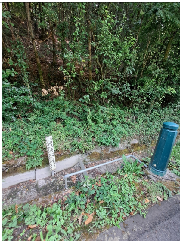
Figure 3 – The flow monitoring point as observed during the visit. No flows from site.
