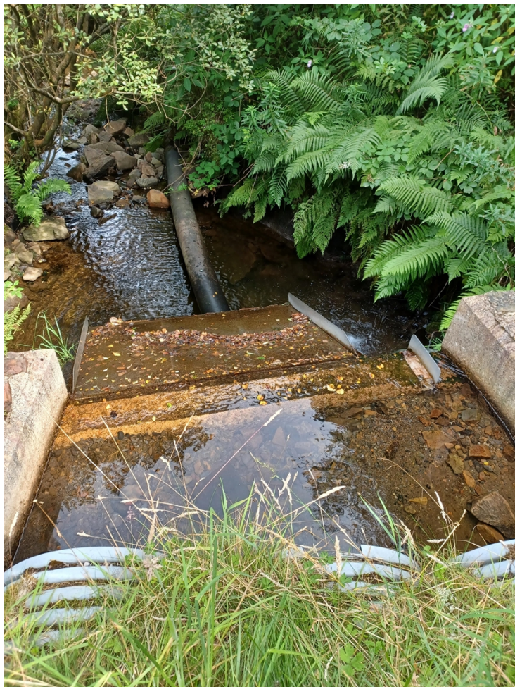
Image 1: Intake structure looking downstream
