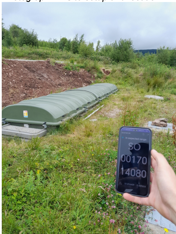
Photograph 1 - Site setup and location
