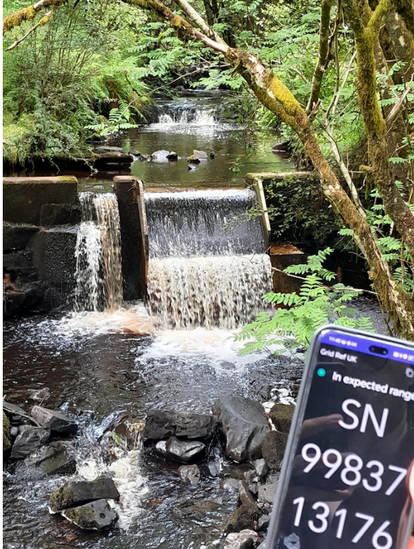
Photograph 1 - location of the intake weir / impoundment
