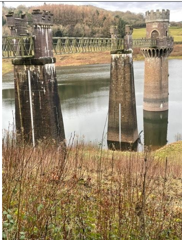
Figure 2: Draw off tower in reservoir
