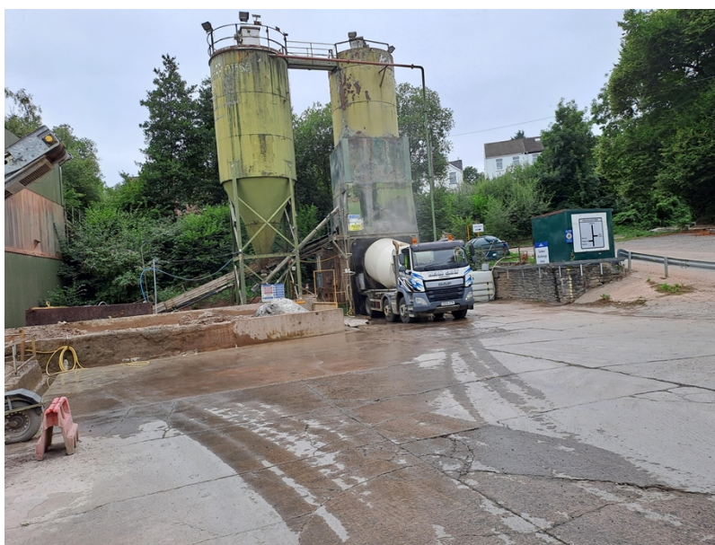
Figure 3 – The site in operation at the time of the visit.
