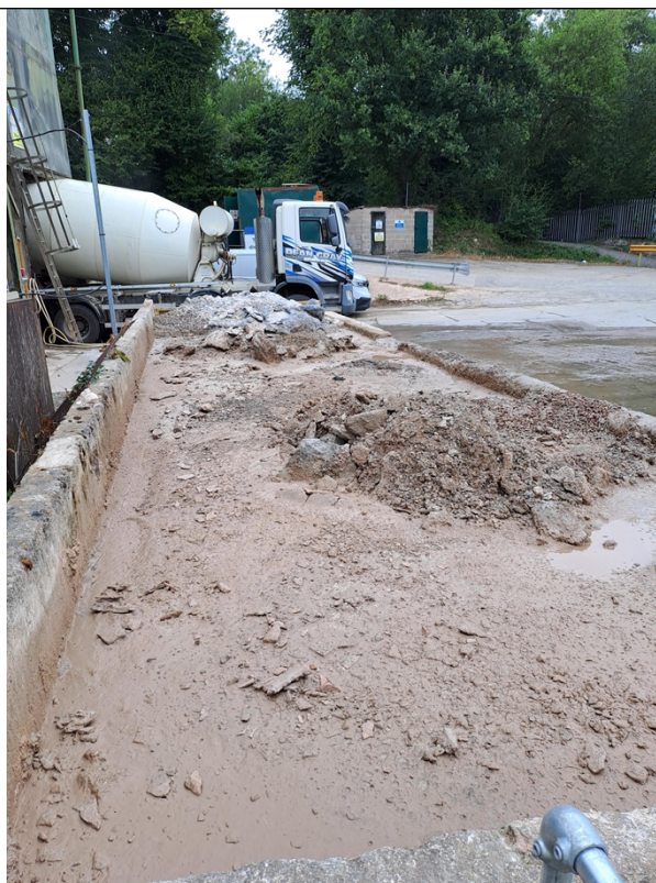
Figure 4 – The wash out pit as observed during the visit.
