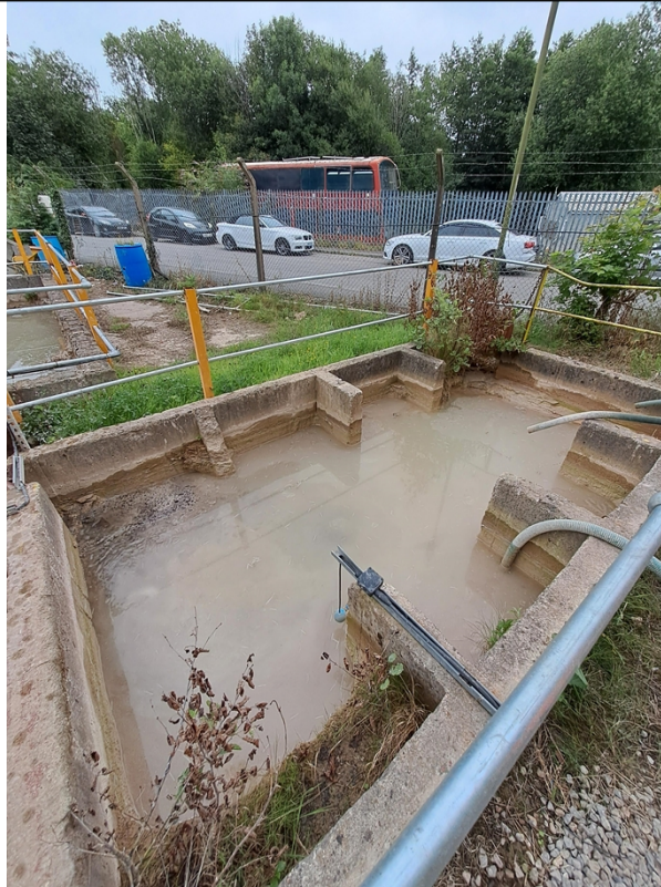
Figure 5 – The primary settlement lagoon as observed during the visit. An active input can be seen in the top left corner from on-site processing.
