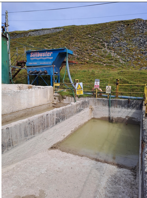
Figure 5 – The end settlement pit and silt buster system as observed during the visit.
