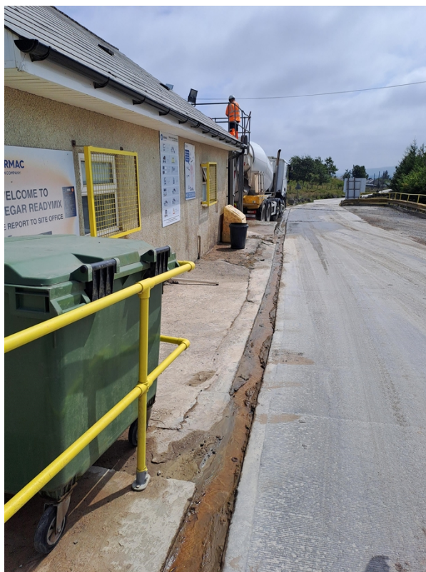
Figure 2 – Water from production flowing through drainage channels towards the settlement pits as observed during the visit.
