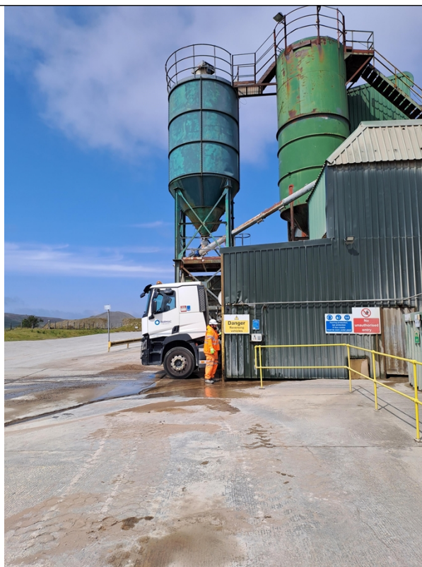
Figure 1 – The production area and water runoff as observed during the visit.
