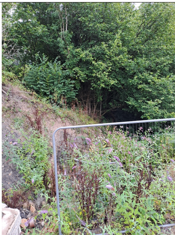
Figure 2 – The discharge point as observed at the time of the visit.
