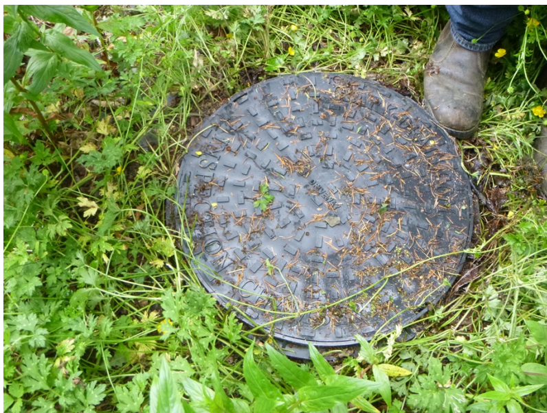
Photograph 2: Final effluent inspection chamber
