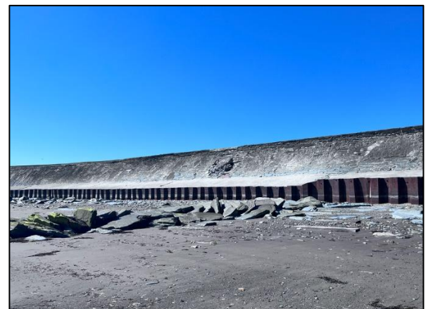
Figure 15: Additional sheet pile protected defence toe.
