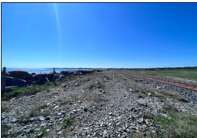
Figure 14: Habitat behind sea wall within rail corridor.
