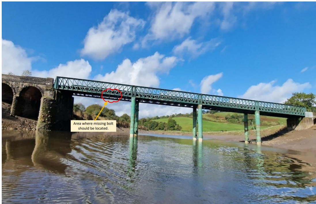
Photo highlighting missing bolt.
