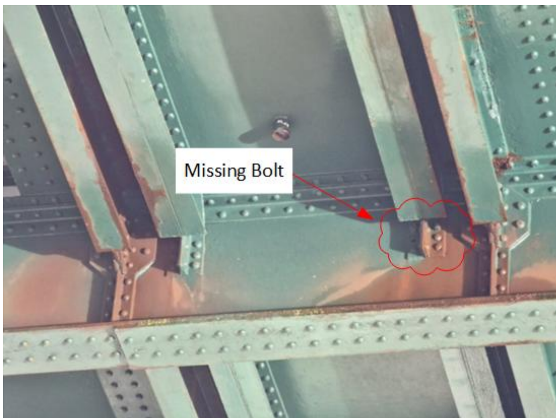
Photo highlighting missing bolt.
