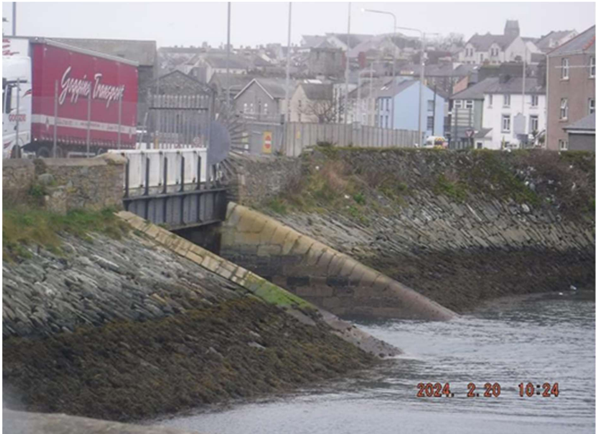
Figure 1. West end of the bridge to Salt Island taken from the north side.
