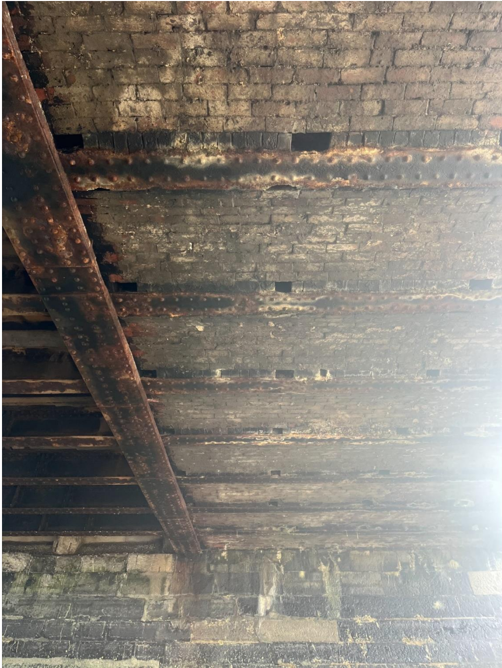
Photograph 7: View of underneath the deck with gaps that could be bat PRF's.
