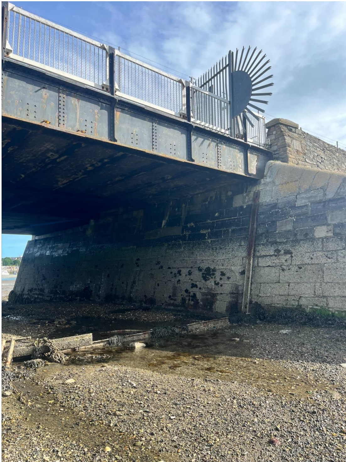
Photograph 4: Viewing facing south-west looking underneath the bridge.
