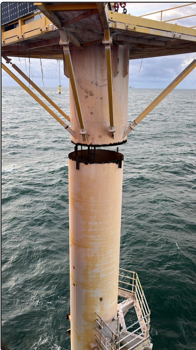
5 Upper platform cut and being lifted.
