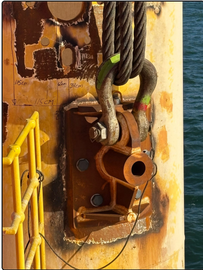
10 Lifting brackets installed.
