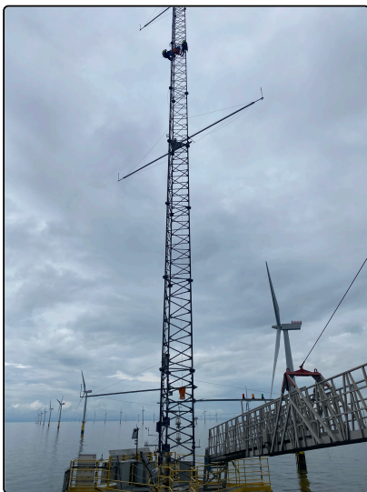
1 Lattice mast prior to removal.
