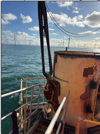
9 Lifting brackets installed.
