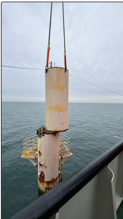
7 Upper monopile section cut from lower monopile section.
