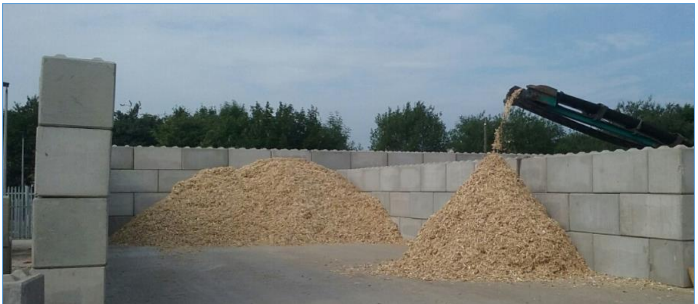
The use of fire walls being used to act as a guard against the spread of fire
