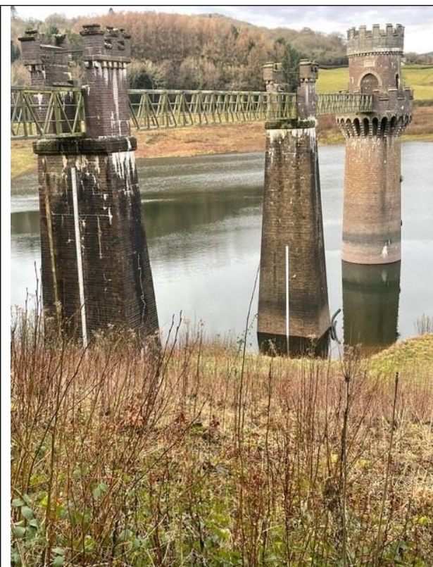
Figure 2: Draw off tower in reservoir
