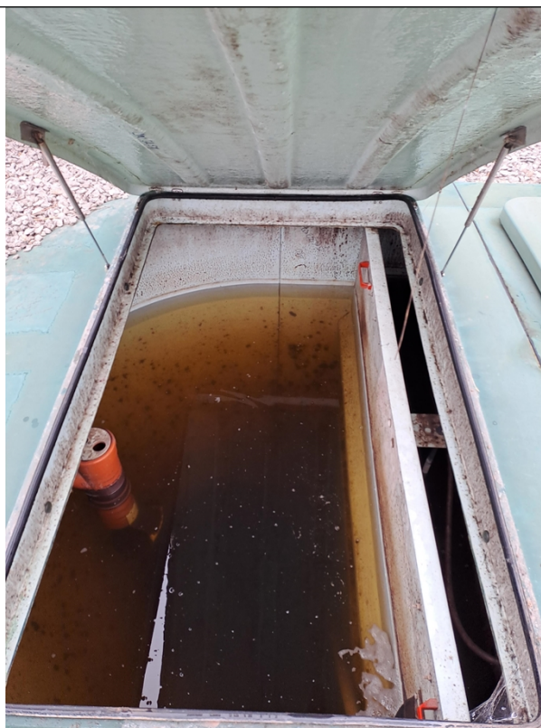
Figure 4 – The final effluent chamber as observed during the visit.
