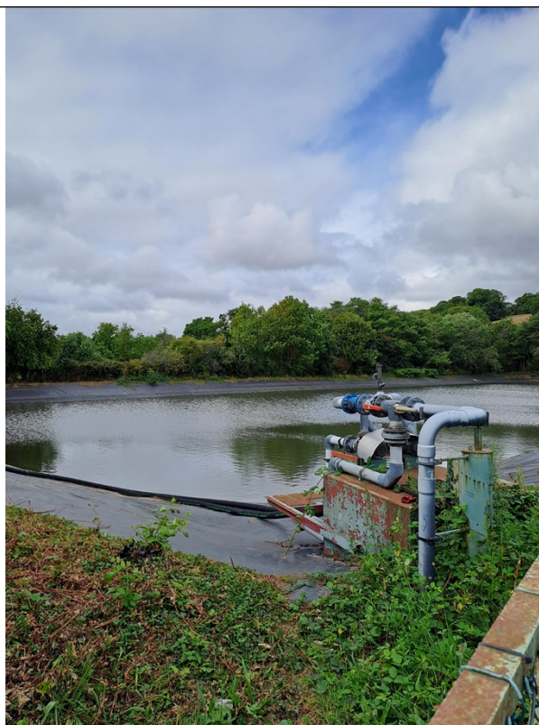
Figure 6 – The reservoir as observed during the visit.
