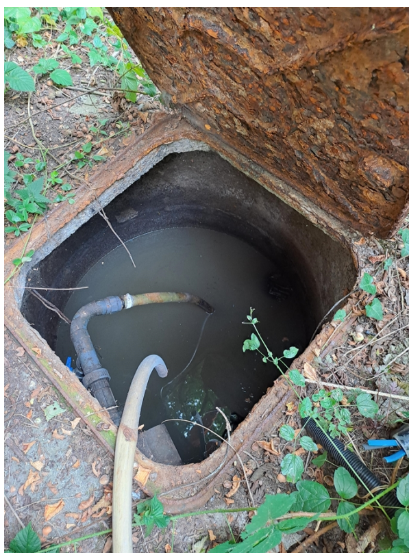
Figure 1 – The primary settlement tank as observed during the visit.
