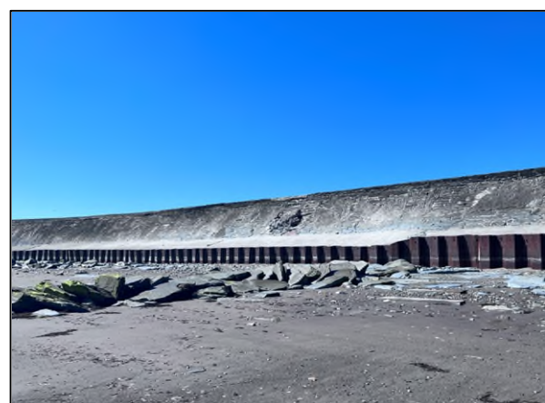
Figure 15: Additional sheet pile protected defence toe.
