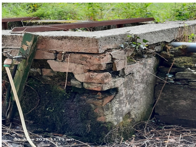
Image 2 – Primary tank in poor disrepair and leaking to ground.
