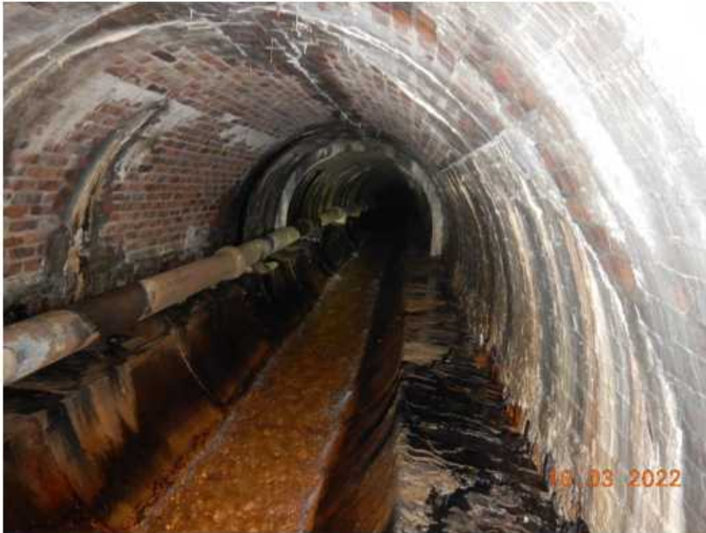
Photo 11 – General view through span 3, looking upstream
