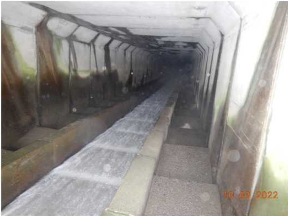
Photo 4 – General view downstream through span 1
