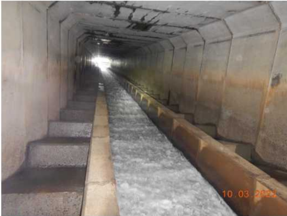
Photo 5 – General view upstream of span 1, taken from Ch54.5m
