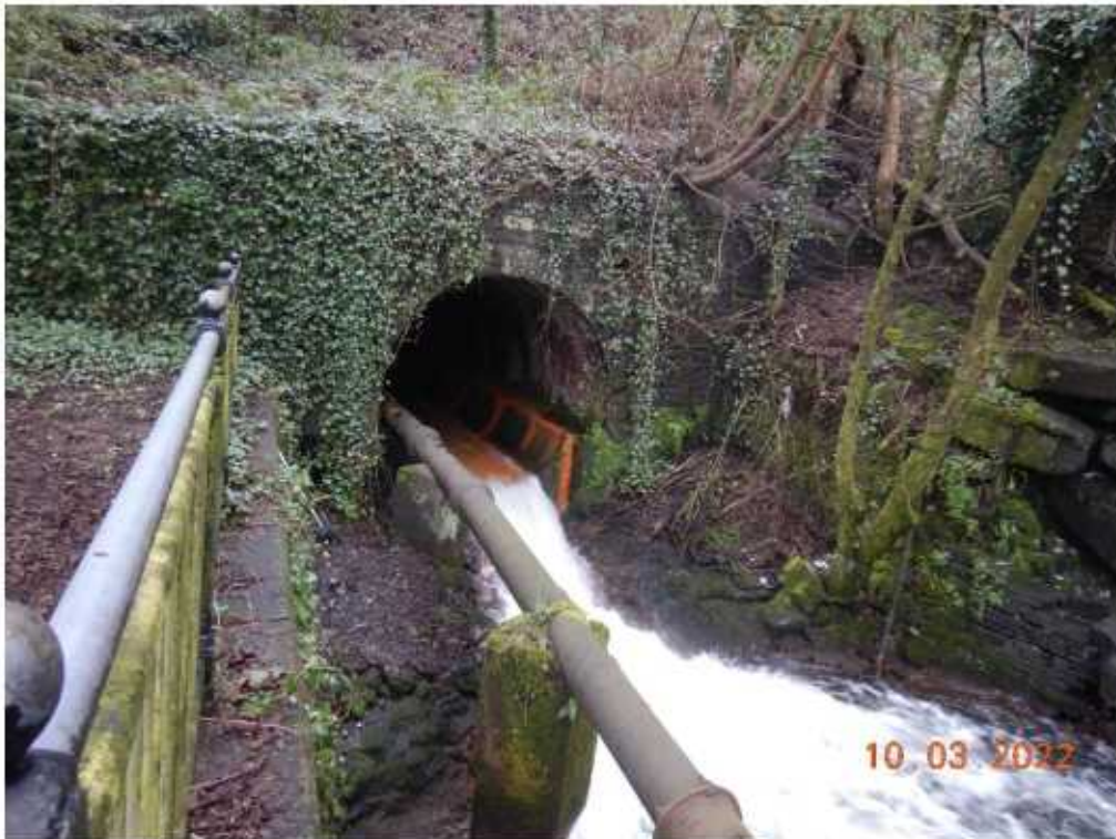
Photo 8 – General view of the culvert outlet
