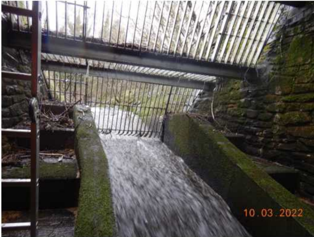
Photo 3 – View upstream from the structure inlet
