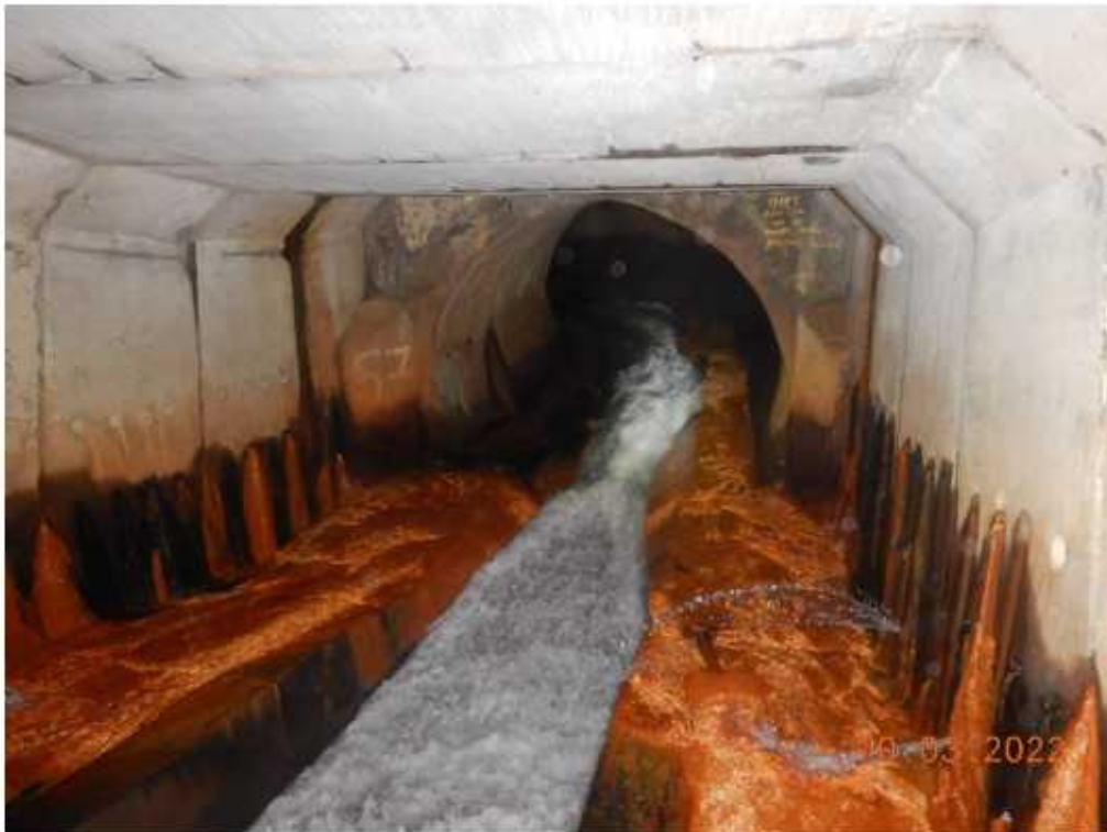
Photo 6 – View of the change in construction to span 2 (CH54.5m)
