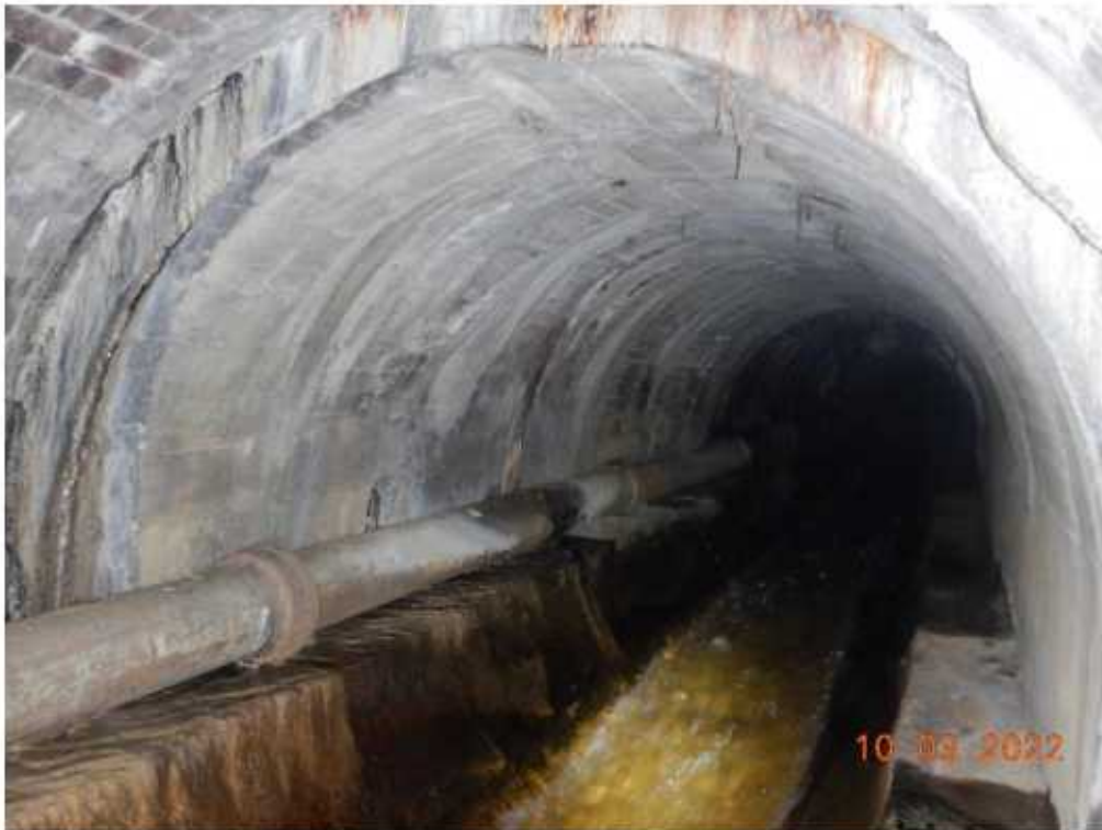
Photo 12 – Example of the cast in situ concrete repairs to the arch
