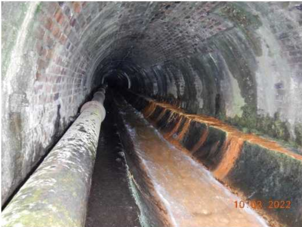
Photo 10 – View upstream of the culvert outlet
