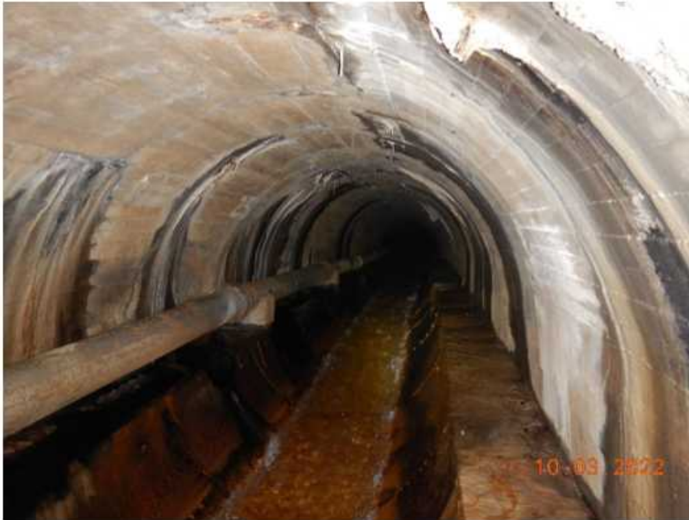
Photo 13 – General view through the cast in situ concrete arch repair sections
