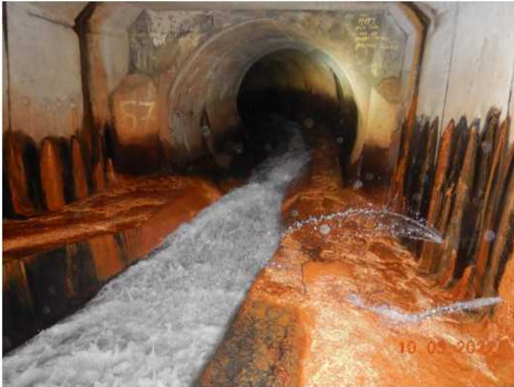
Photo 7 – View through span 2, looking downstream from Ch54.5m)
