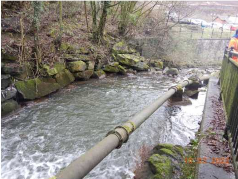
Photo 9 – View downstream from the culvert outlet
