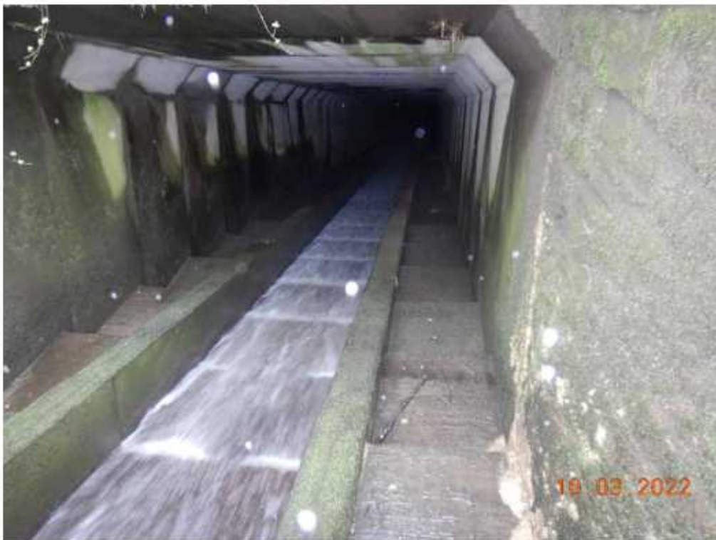
Photo 2 –View downstream from the structure inlet
