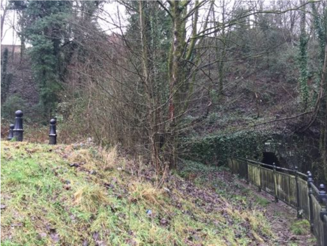
Photo E3: SS 99161 92694. View of proposed turbine house location (to the left, by the bollards) and the route of the proposed tailrace to the discharge point where the culvert outflow is located.
