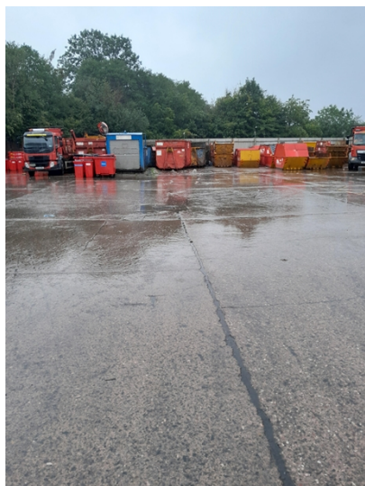
Fig 1. (overview of site)
