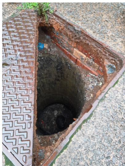
First Interceptor Chamber (Fig 3)
