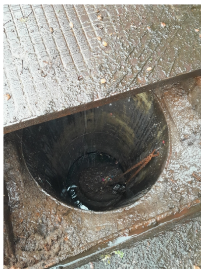
Final Interceptor chamber (Fig 4)
