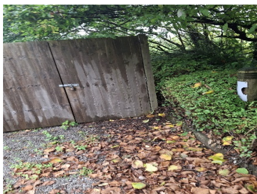
Figure 2: Access point to the system w/ padlocked door
