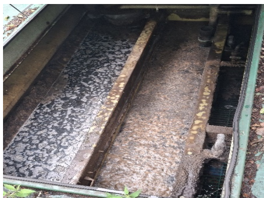
Figure 8: Third chamber with turbid water and high solid waste carry over
