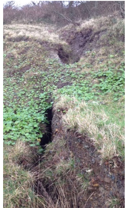
cut-off drains collecting surface water. This water is able to percolate deeper into the slope.
