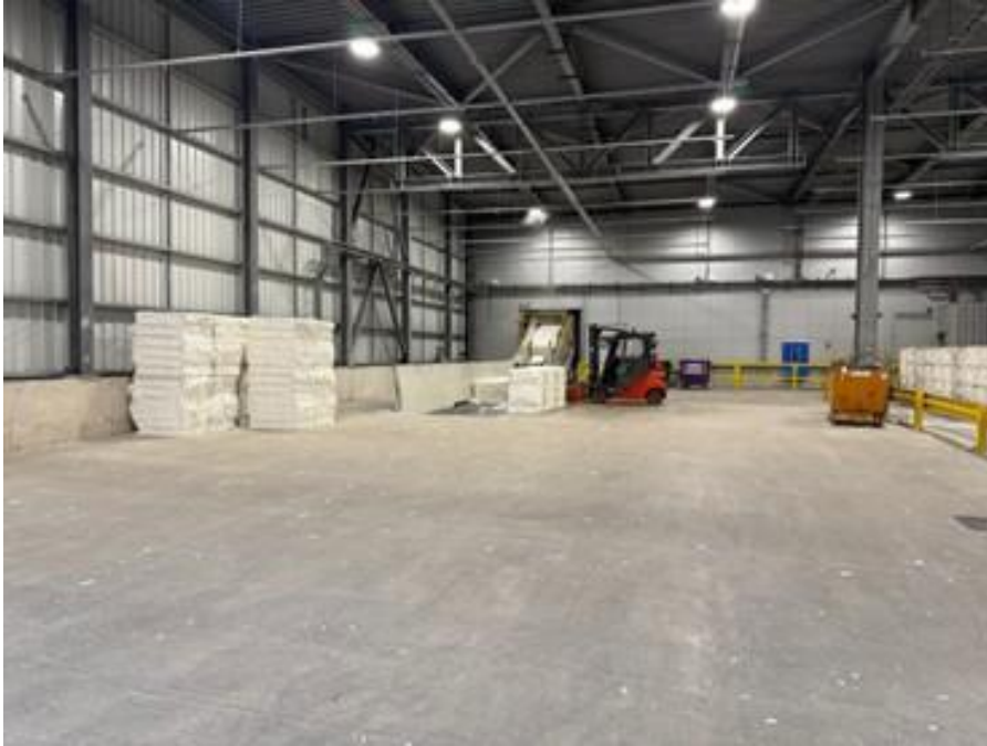
Photograph 10-1: Surfacing within the broke storage area
