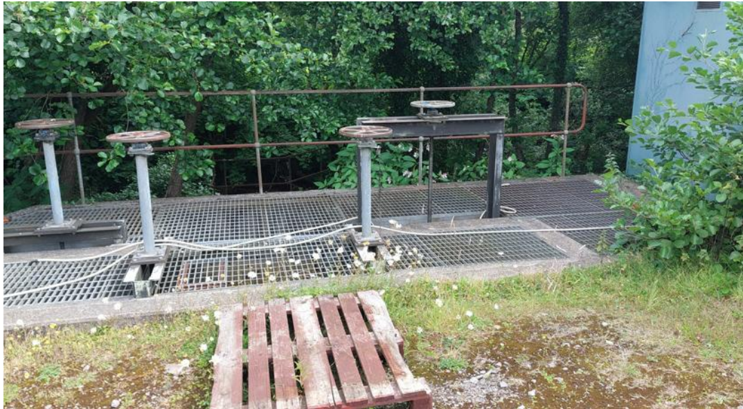
Photograph 10-4: Effluent outfall diversion chamber
