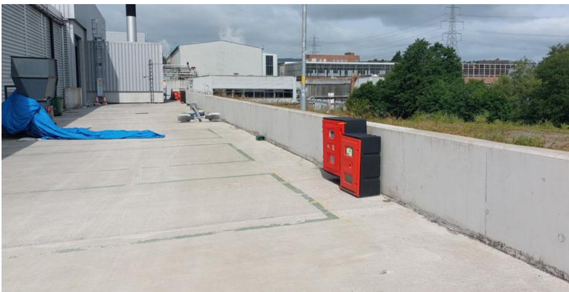
Photograph 10-2: Department A retaining wall
