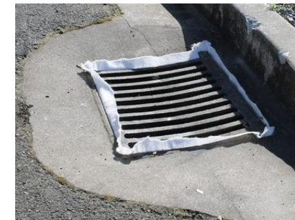
Fig.3.15 – gully silt sock
