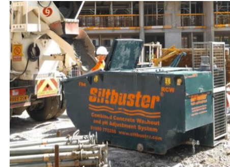
Fig.3.13 – Proprietary concrete wash out facilities
