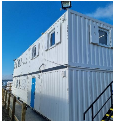
Fig.4.1 – Typical Site Accommodation
