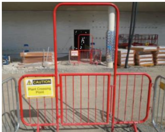
Fig.4.3 –Example crossing point
