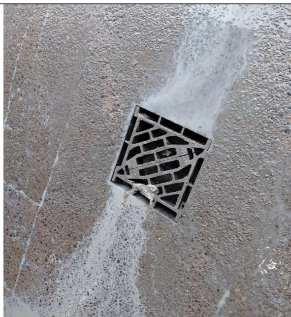
Photo 4 Free flowing drain on operational side of the site
