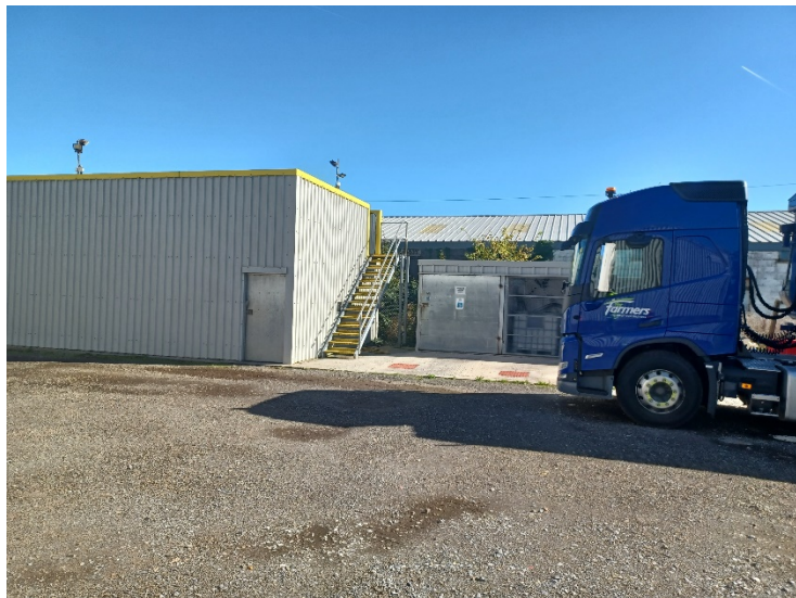
Photo above showing Lorry Wash area and bore hole extraction point
