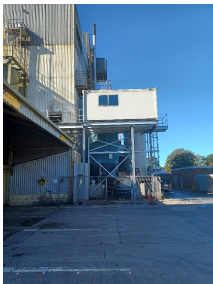
Photo above showing newly constructed control room.
