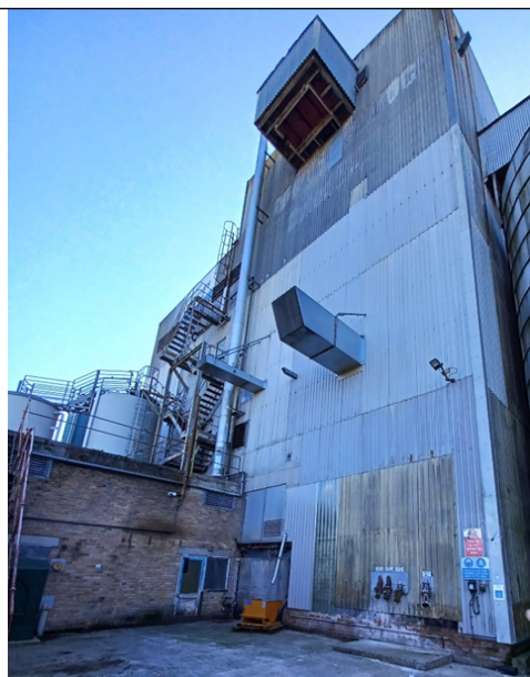
Photo above showing grinder extraction points.
