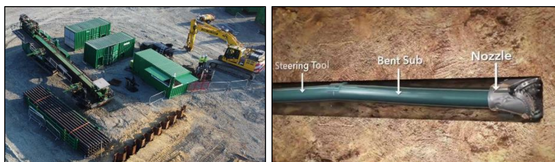
Figure 4.10: Typical drilling rig and pilot drilling assembly
