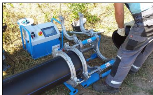
Figure 4.8: Typical pipe welding equipment, storage of pipes and welfare not shown
