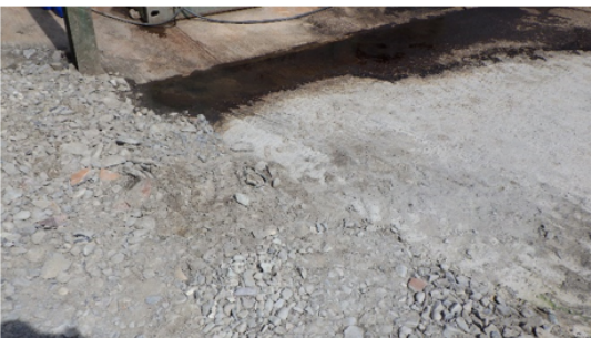
Photograph 12. Runoff of leachate to ground around the leachate treatment plant.
