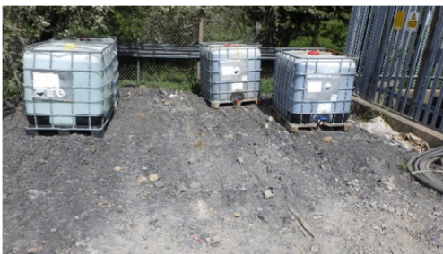
Photograph 8. IBC containing Ferric Chloride and Sodium Hydroxide stored on permeable base
