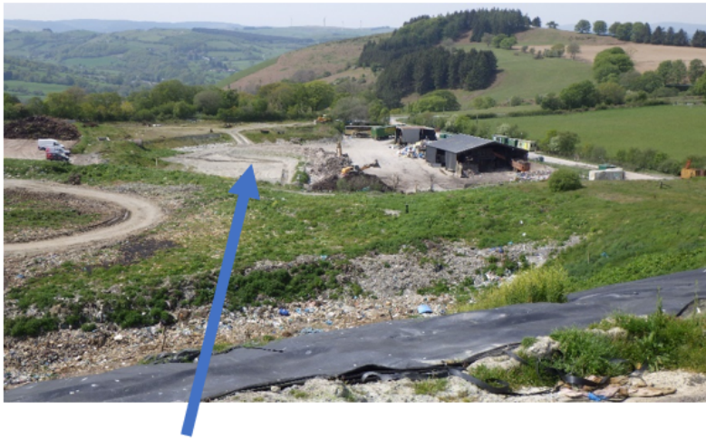
Photograph 2 – Previous area that was ponding with contaminated waste now dry.
