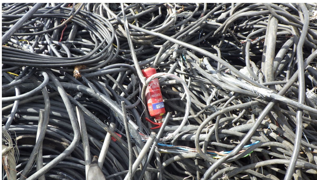
A fire extinguisher in a pile of cables.
