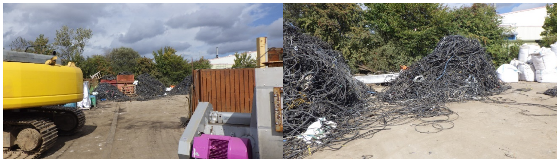
Cables stored on site
