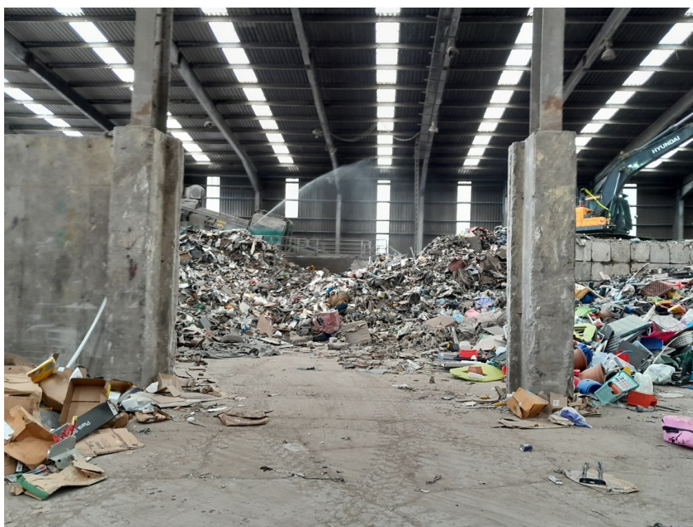
Photo 2 - View inside waste transfer station building
