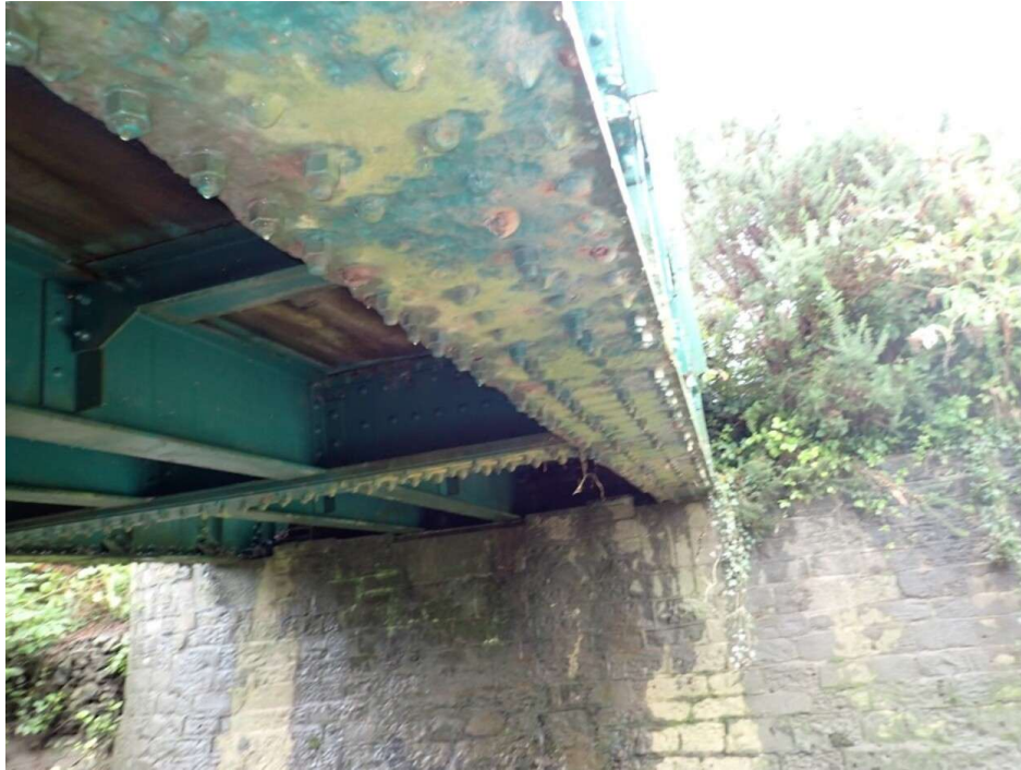
Photo 15: Main Girder 2 Bottom Flange (28/08/2024)
