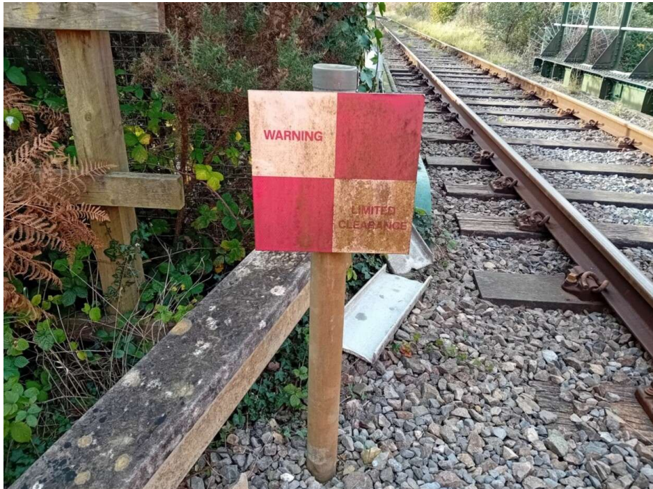
Photo 36: Typical Limited Clearance Plate (12/11/2024)
