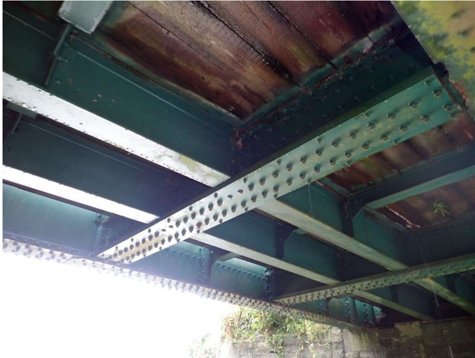
Photo 19: HM Cross Girder (28/08/2024)
