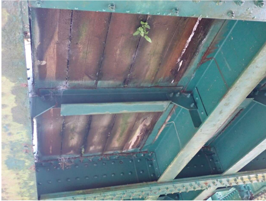
Photo 21: Typical Deck Boards (28/08/2024)
