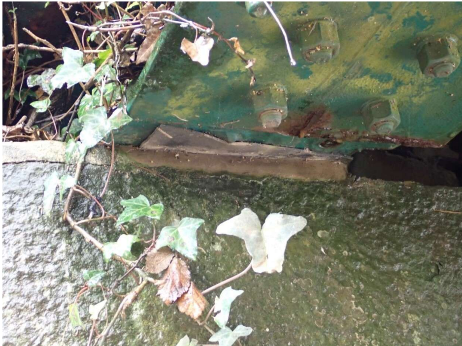
Photo 30: Lead Bearing (28/08/2024)
