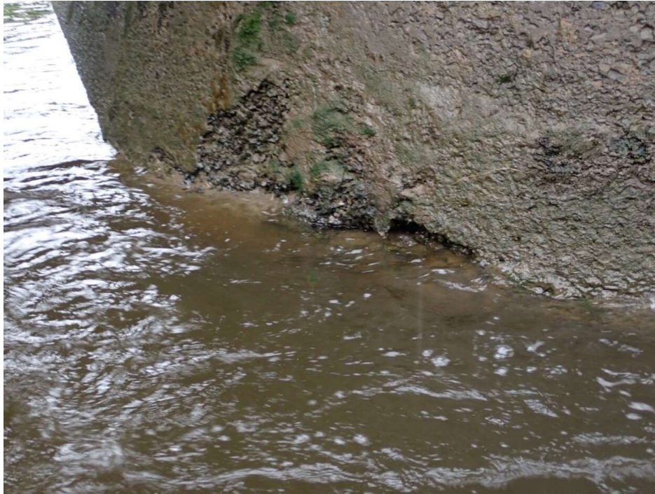
Photo 23: Spalling (28/08/2024)
