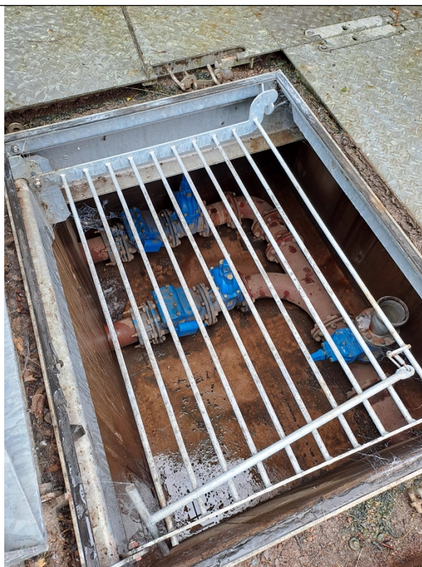
Figure 3 – The valve chamber as observed during the visit.
