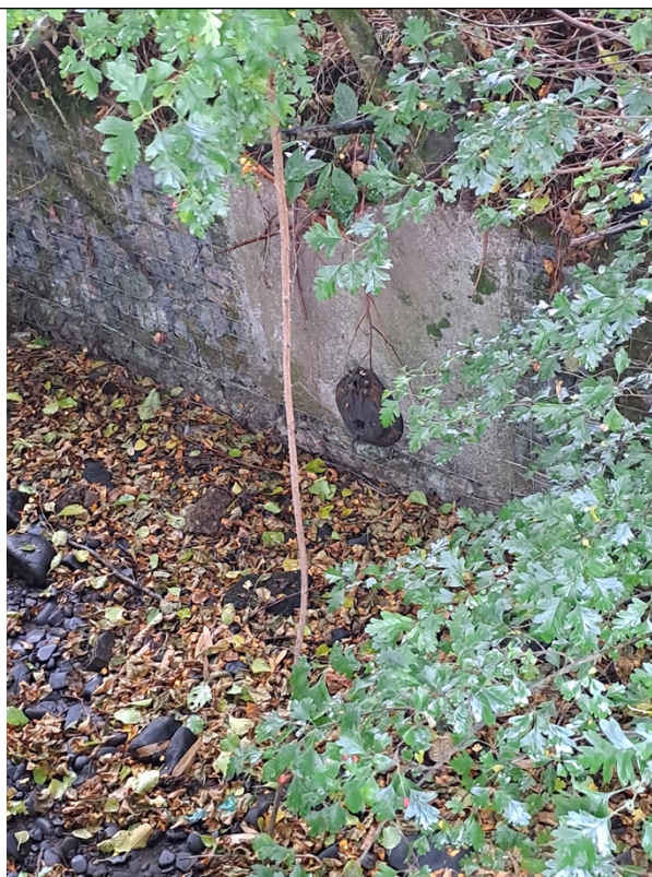
Figure 8 – The EO discharge point located at ~ ST1458393248 as observed during the visit.
