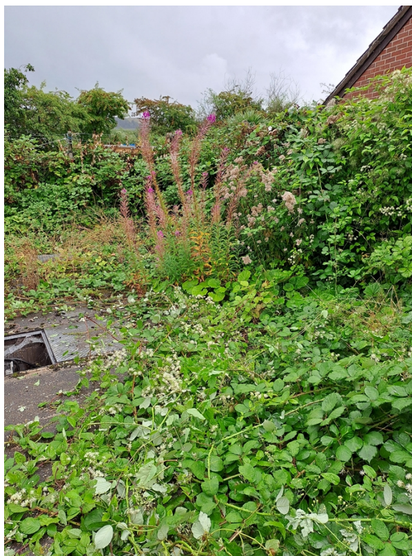
Figure 1 – Heavy vegetation growth within the SPS compound as observed during the visit.
