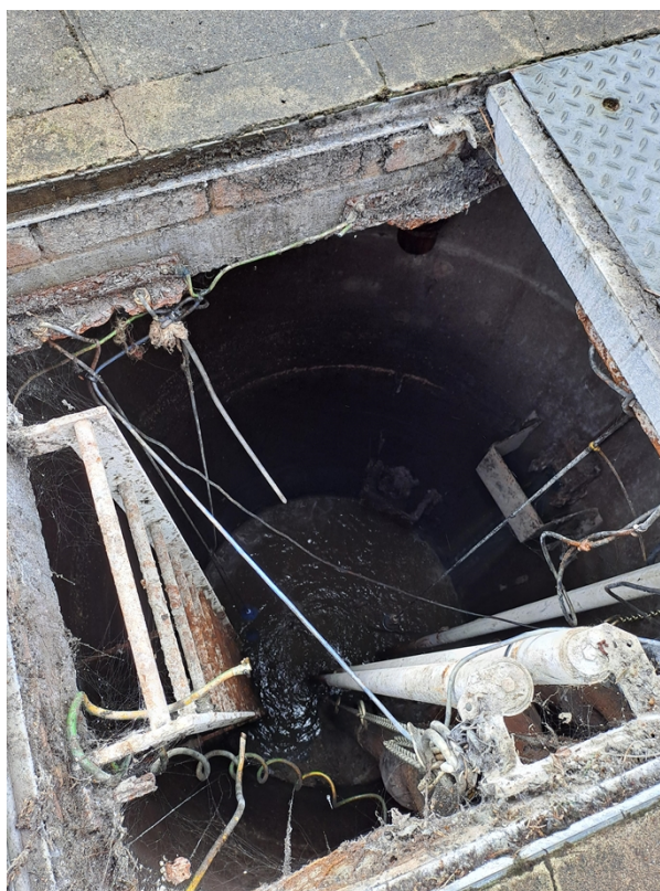
Figure 2 – The wet well as observed during the visit.
