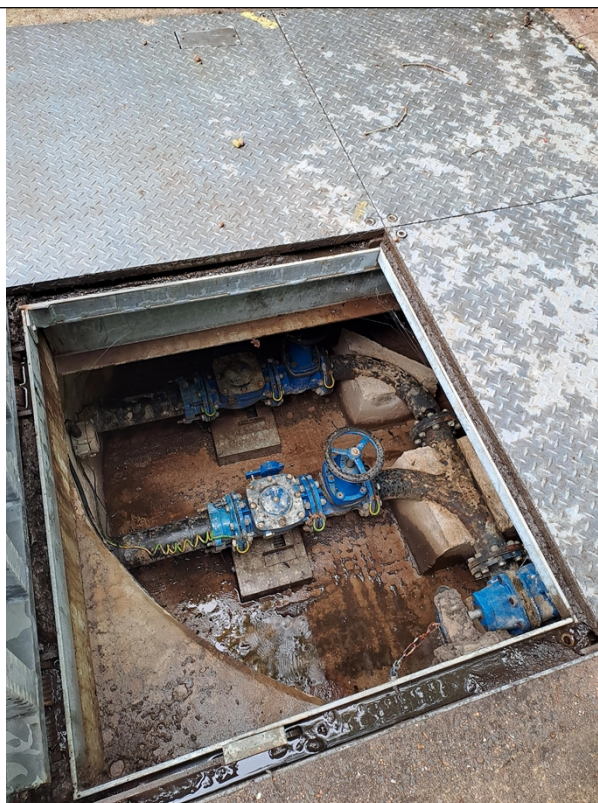
Figure 4 - The valve chamber as observed during the visit.
