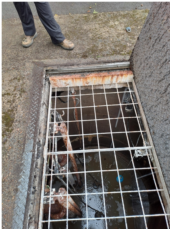
Figure 2 – A view of the wet well as observed during the visit. The discharge outlet can be see with the 10mm screen in place.
