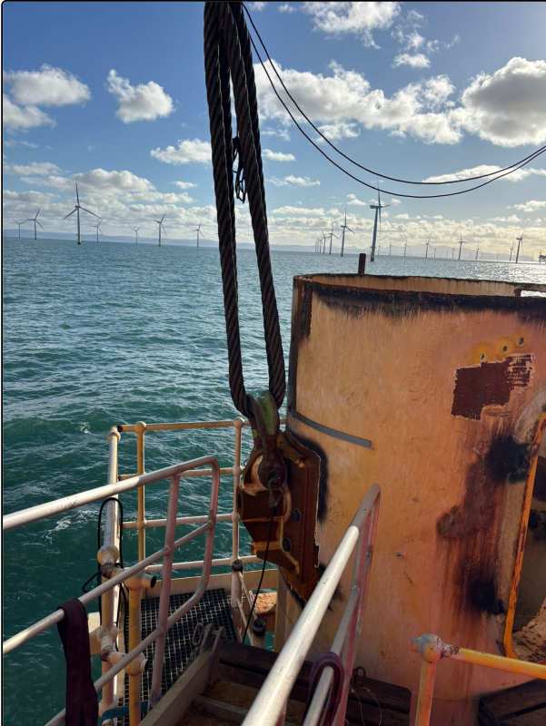
9 Lifting brackets installed.
