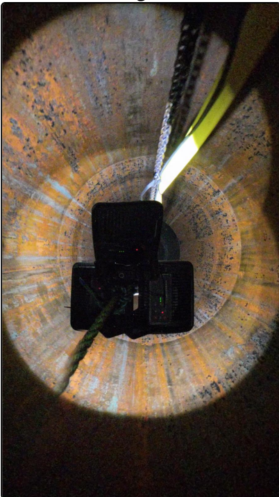
12 Camera and Lights being lowered into the monopile.
