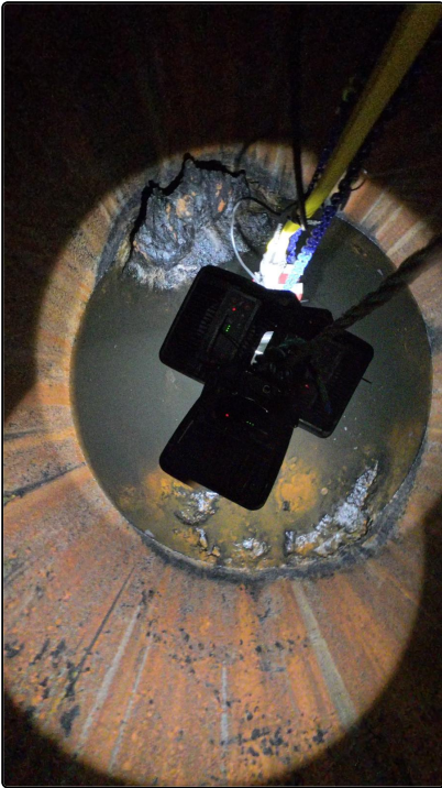
13 Camera and Lights at the bottom of the monopile.
