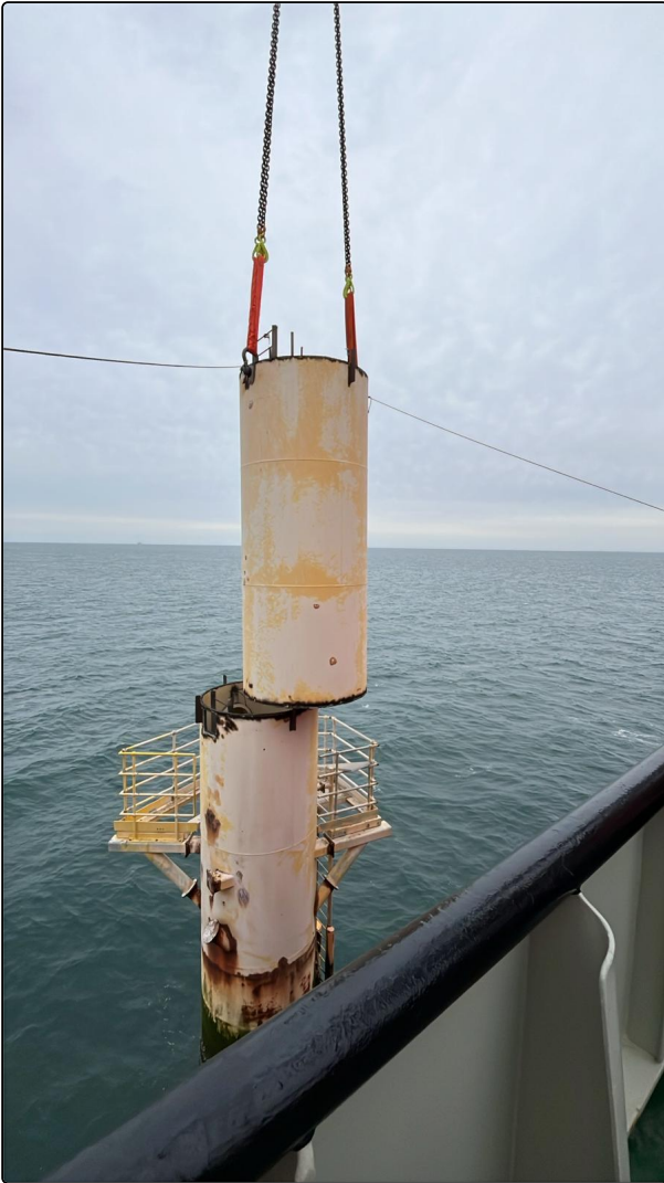
7 Upper monopile section cut from lower monopile section.
