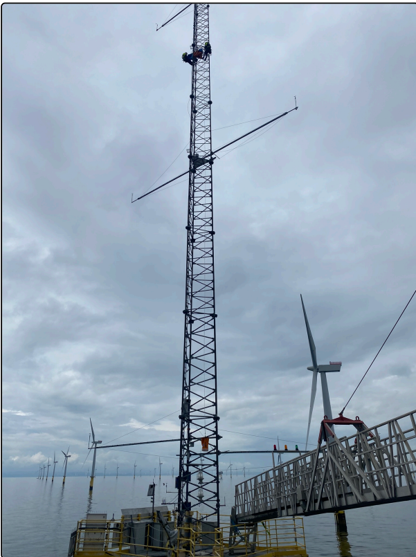
1 Lattice mast prior to removal.
