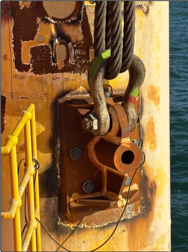
10 Lifting brackets installed.
