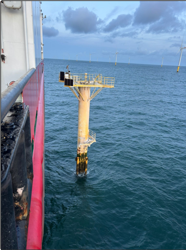
3 WIND SERVER arriving to the Gwynt Y Mor Meteorological Mast
