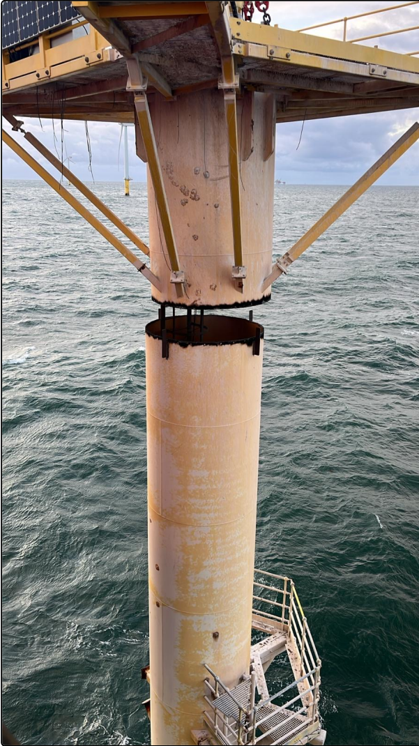
5 Upper platform cut and being lifted.
