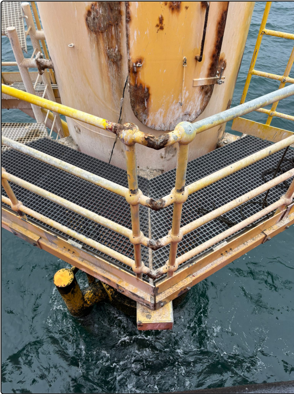
8 Access platform with new grating installed. Serving as working area.
