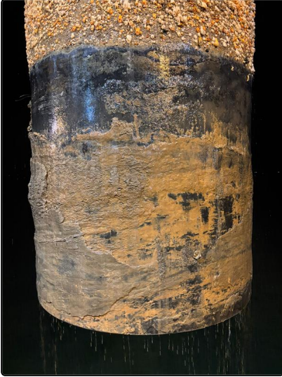
15 MP being lifted out of the water
