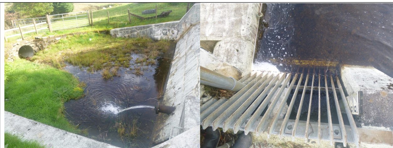
Figures 7 & 8: Orifice Plate and Abstraction Screen at Nant y Bog
