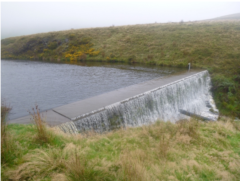
Figure 1. The intake weir on the Nant Rhyd.
