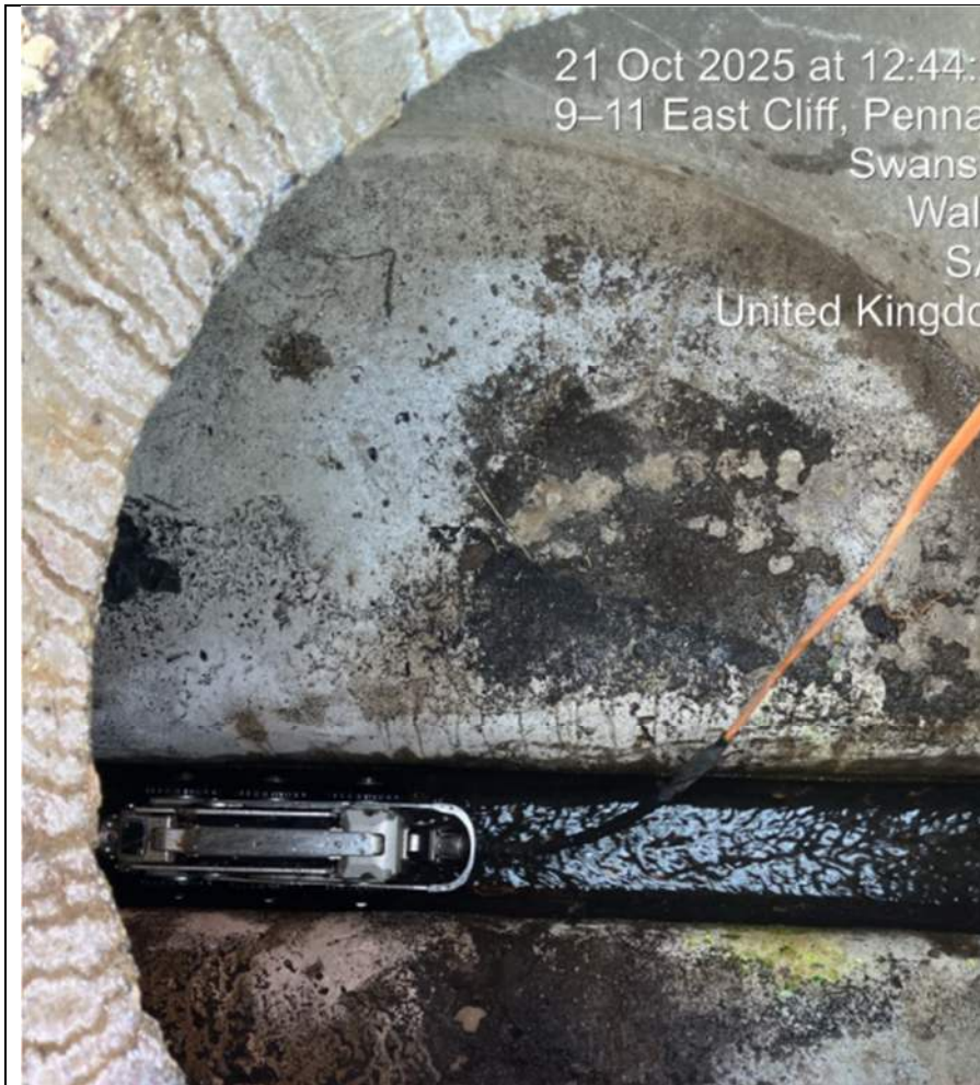
Uncharted m/h on grass verge next to Eastcliff Rd
