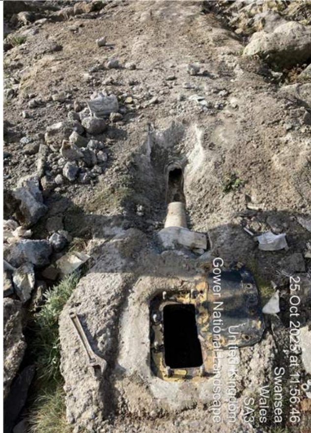
Excavation on FE line.
