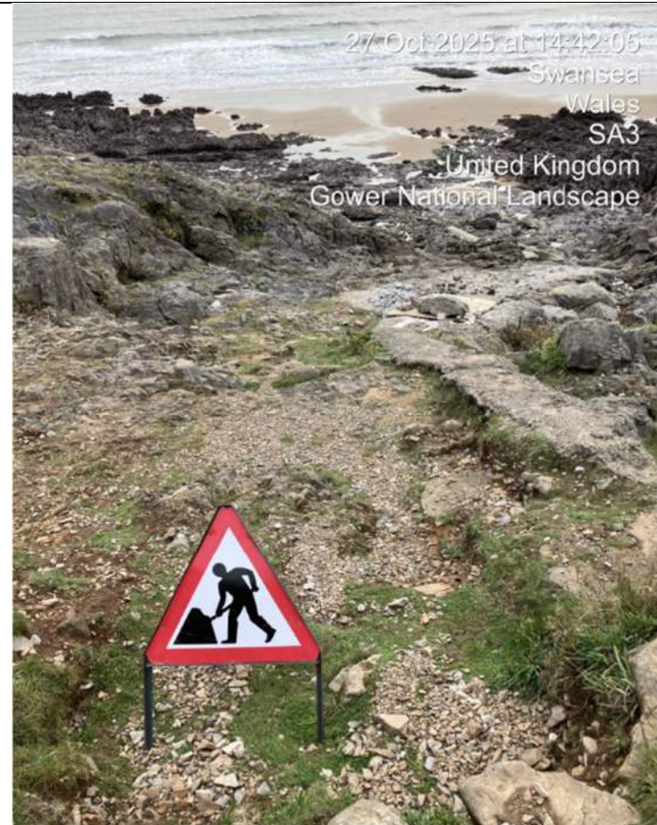
Temporary repair to contain flow
