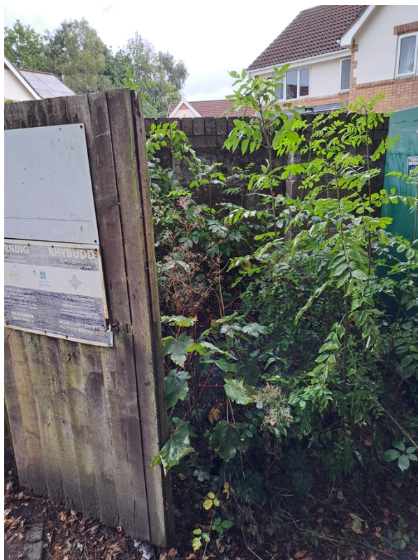
Figure 2 – Site conditions as observed during the visit.
