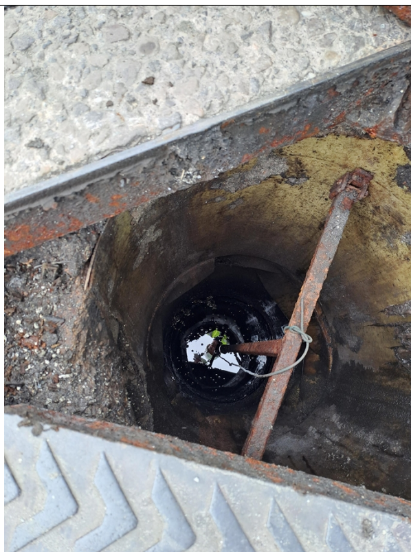
Figure 2 – The oil interceptor as observed during the visit.
