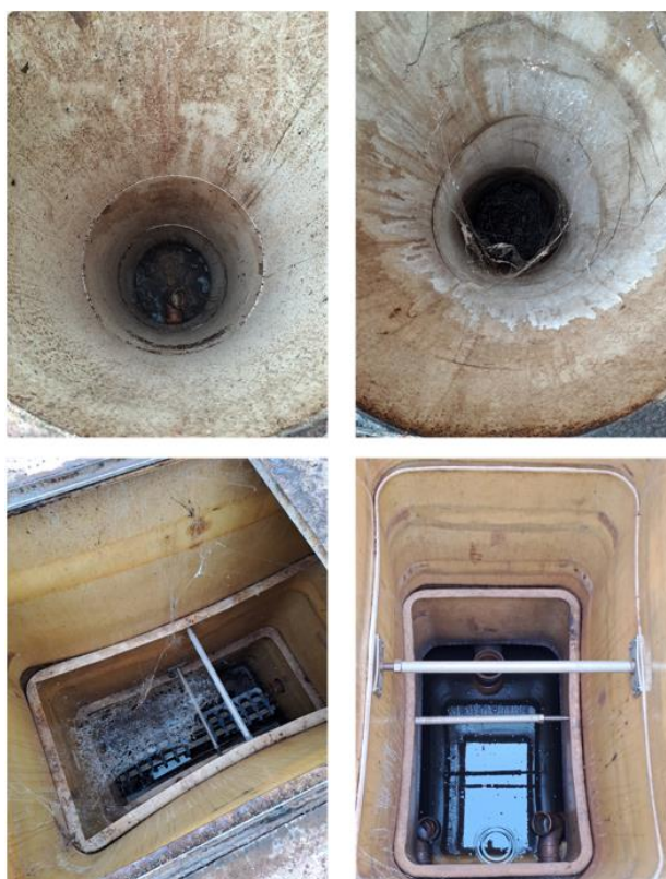
Figure 6 – The effluent chambers as observed during the visit.
